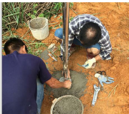
Ground lead operation
