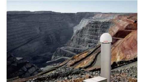
Tailings pond Monitoring
