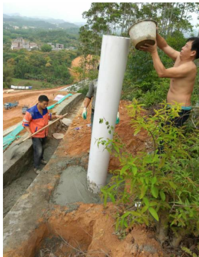
Pouring of displacement observation pillar
