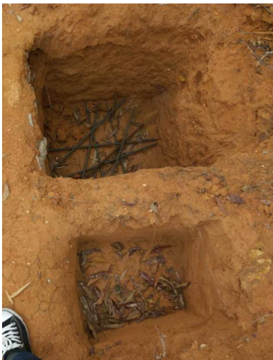
Foundation pit of displacement observation pillar
