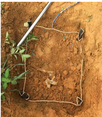
Lightning protection construction
