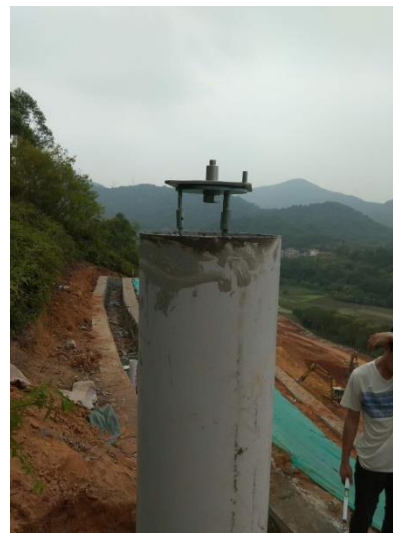
Displacement observation pillar pouring completion
