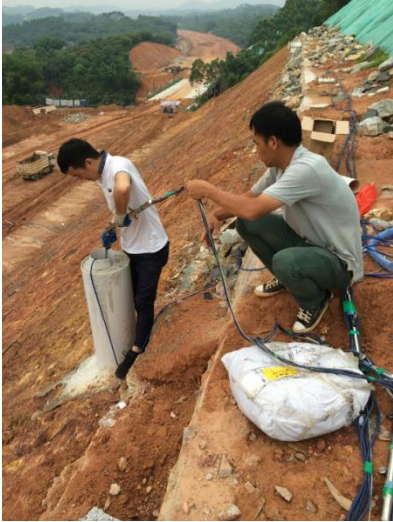
Inclinometer installation
