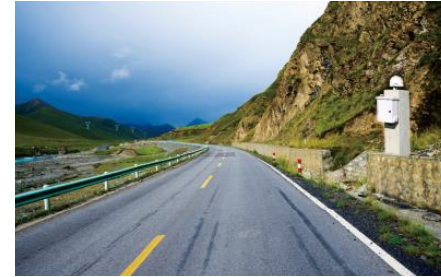
Road Slope Monitoring
