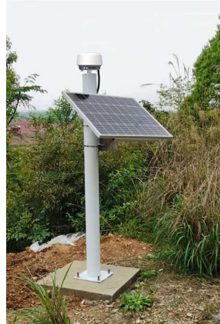
Install on disaster site
