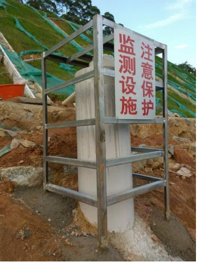
Completion of Inclinometer installation
