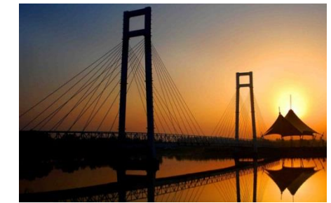
Bridge health Monitoring
