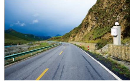
Road Slope Monitoring
