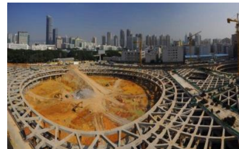
Foundation Pit Monitoring
