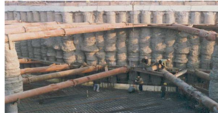
Drilled filling pile
