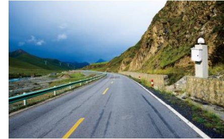
Road Slope Monitoring
