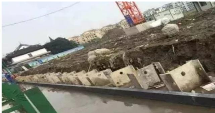
Soil Mixing Wall
