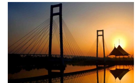
Bridge health Monitoring
