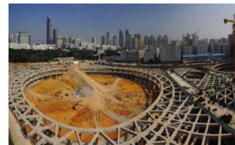
Foundation Pit Monitoring
