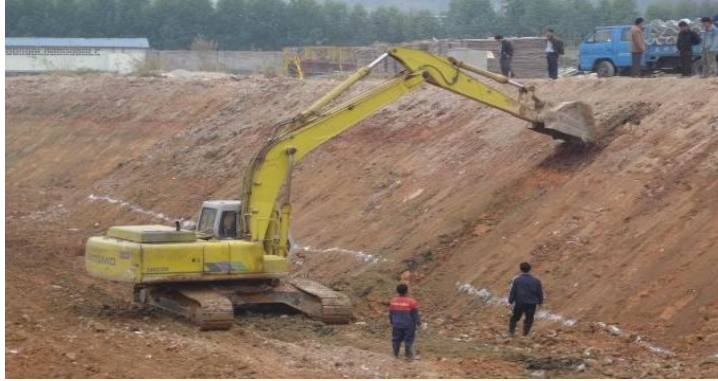
Step-slope excavation
