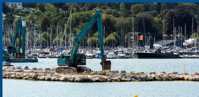
Port and Wharf Construction
